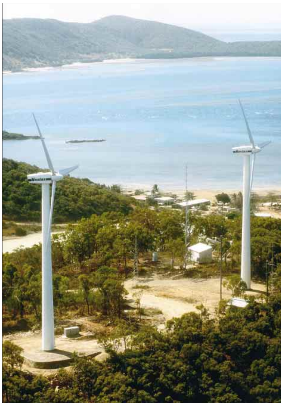
The wind turbines on Milman Hill, Thursday Island.
