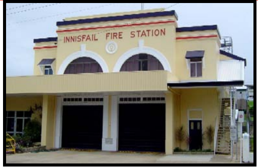
Innisfail Fire Station
