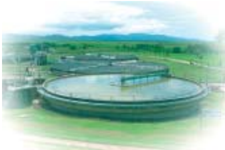
Primary Settling Tank
